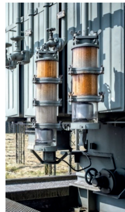
Conventional dehydrating breathers with color change from orange to colorless
