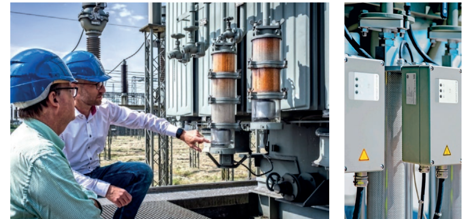
Comparison of a conventional (left) and a maintenance-free dehydrating breather (right).
